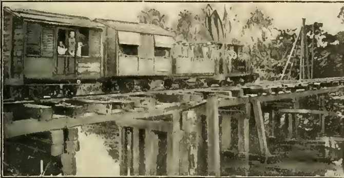
WORKMAN'S TRAIN CROSSING TEMPORARY TRESTLE.
